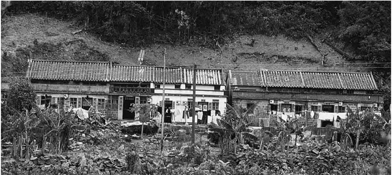
In South China attached houses are built of cement and have tiled roofs, and at the New Year they all display traditional decorations. Paintings and calligraphy honor the Kitchen God and other auspicious guardians who will keep the evil spirits away from the door. PHOTO BY JOAN LEBOLD COHEN.
